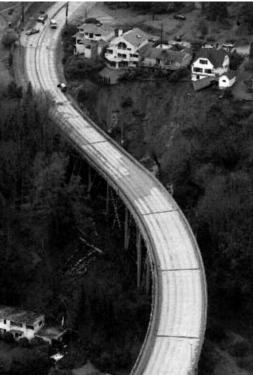
The January 1997 mudslide swept down the hill between two of the bridge's support columns, knocking out cross braces and filling the Navy home below the bridge with debris. Courtesy of The Seattle Times.
