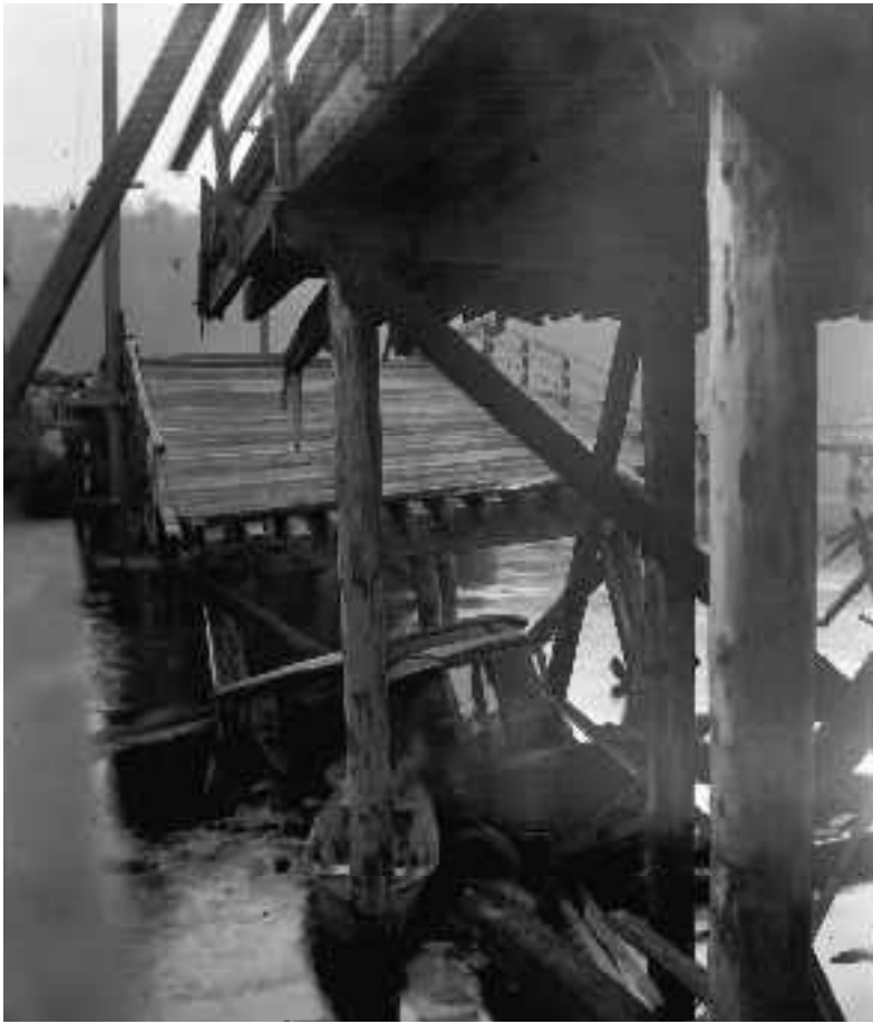
Getting to and from Magnolia wasn't always easy. The license plate of this unfortunate vehicle dates this photo at 1925. Rotted timbers were likely the cause of the trestle's collapse. Museum of History and Industry #83.10, 368.2.
