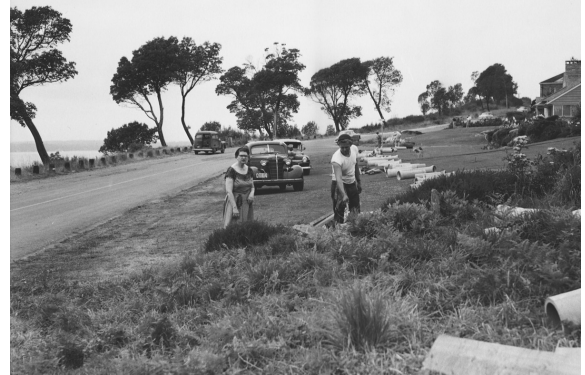
Straight stretch paved and landscaping being added Seattle City Archive c1953
