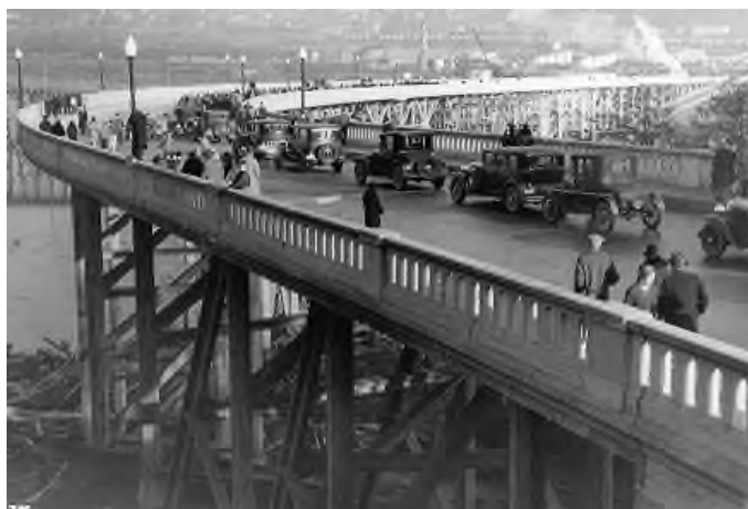
The West Garfield Street Bridge opened to vehicles and pedestrians in December 1930. This photo was taken from the west end of the Bridge. Photo courtesy of Seattle Engineering Department #458
