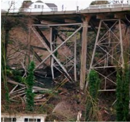
This is a view of secondary supports built for increased earthquake protection on the Magnolia Bridge in Seattle that was destroyed Thursday by a mud slide. The road is the main access to the Magnolia area and may be closed for some time. The mud slide also damaged the home below the Bridge that is owned by the Navy [The Admiral's House]. (AP Photo/Loren Callahan/seattlepi.com file)
